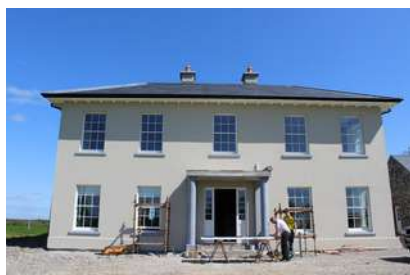
New windows and doors
